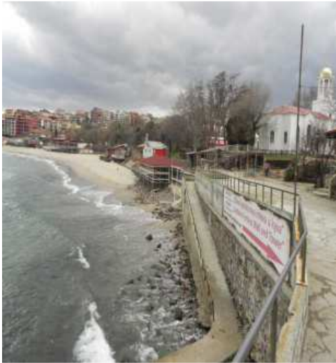
Ramp for people with disabilities to the Central Beach
