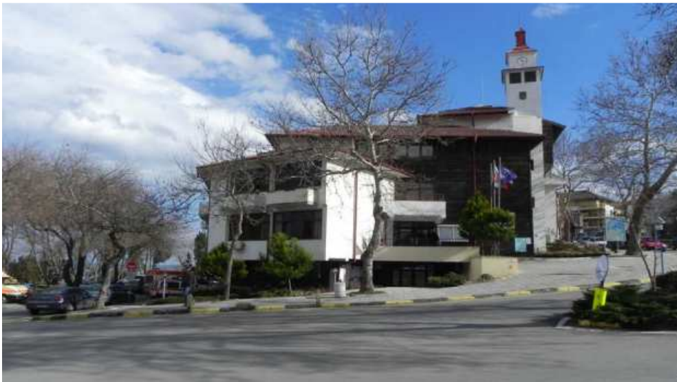
Building of the Municipal Administration, located at the beginning of Archaeological Reserve Ancient Town of Apollonia
