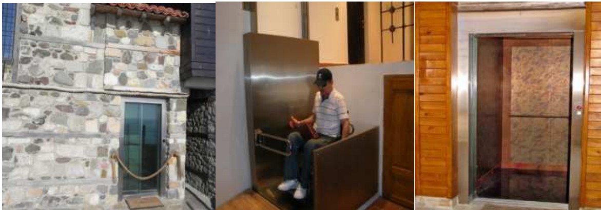
The construction of a lift and a platform
